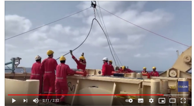
EllaLink EllaLeaks STE11 - Final Splice
